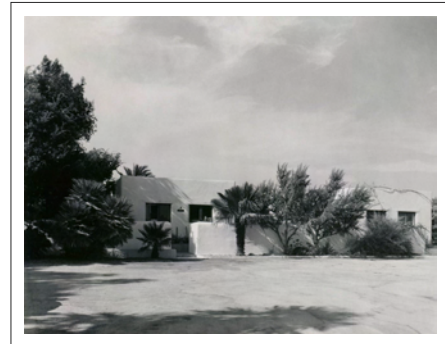
This Pueblo style stucco building made of thick adobe was the office.
