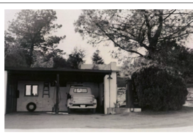
Across and down the road from where the Sandersons lived, is the building with the tool shop and garage.
